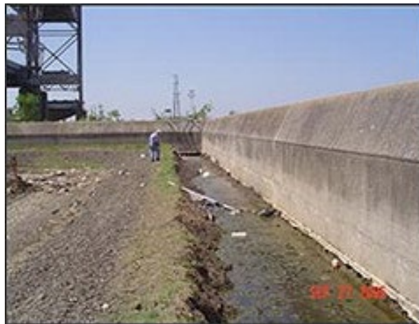
Figure 2-12: Effects of Scour on a Levee and Floodwall Near the IHNC
